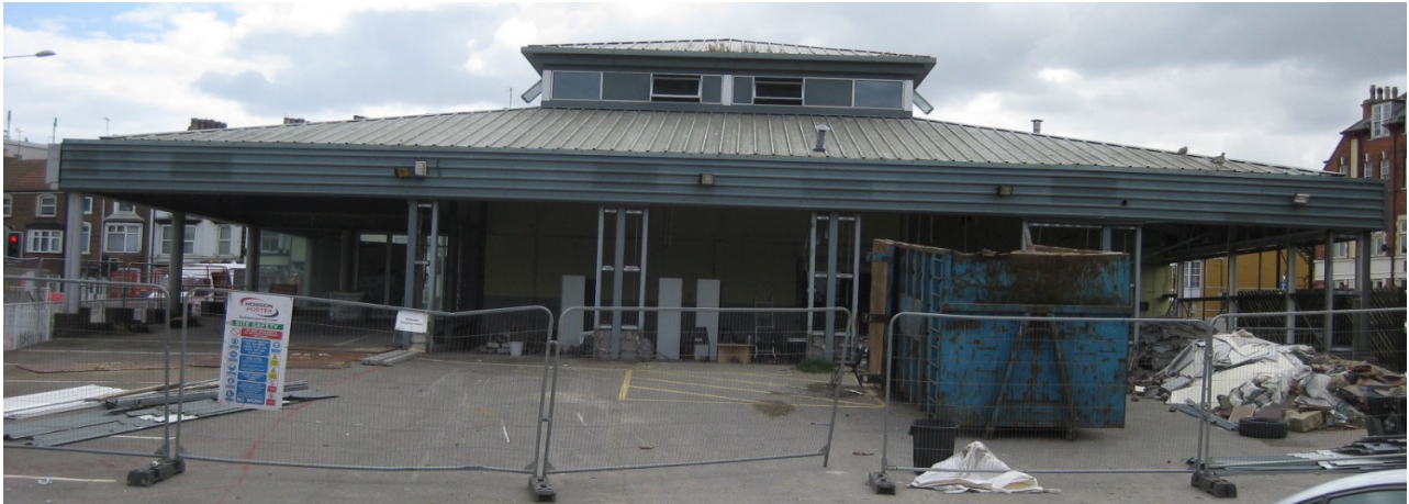
Springfield House ready for demolition
