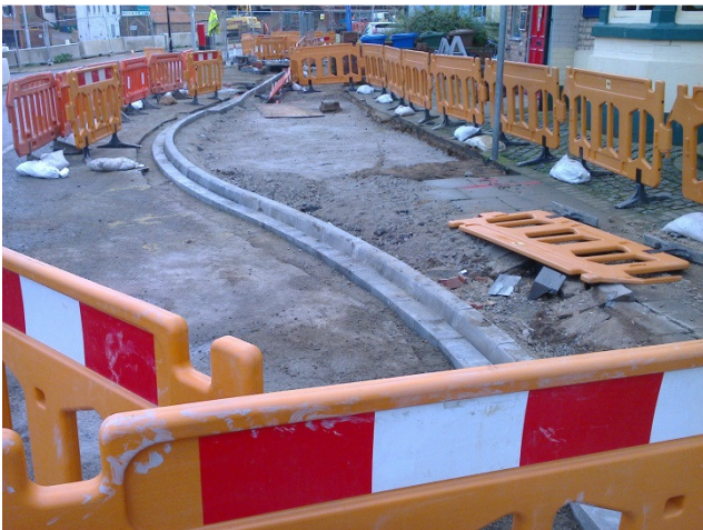
Kerbing, channel, drainage and paving works Hilderthorpe Road
