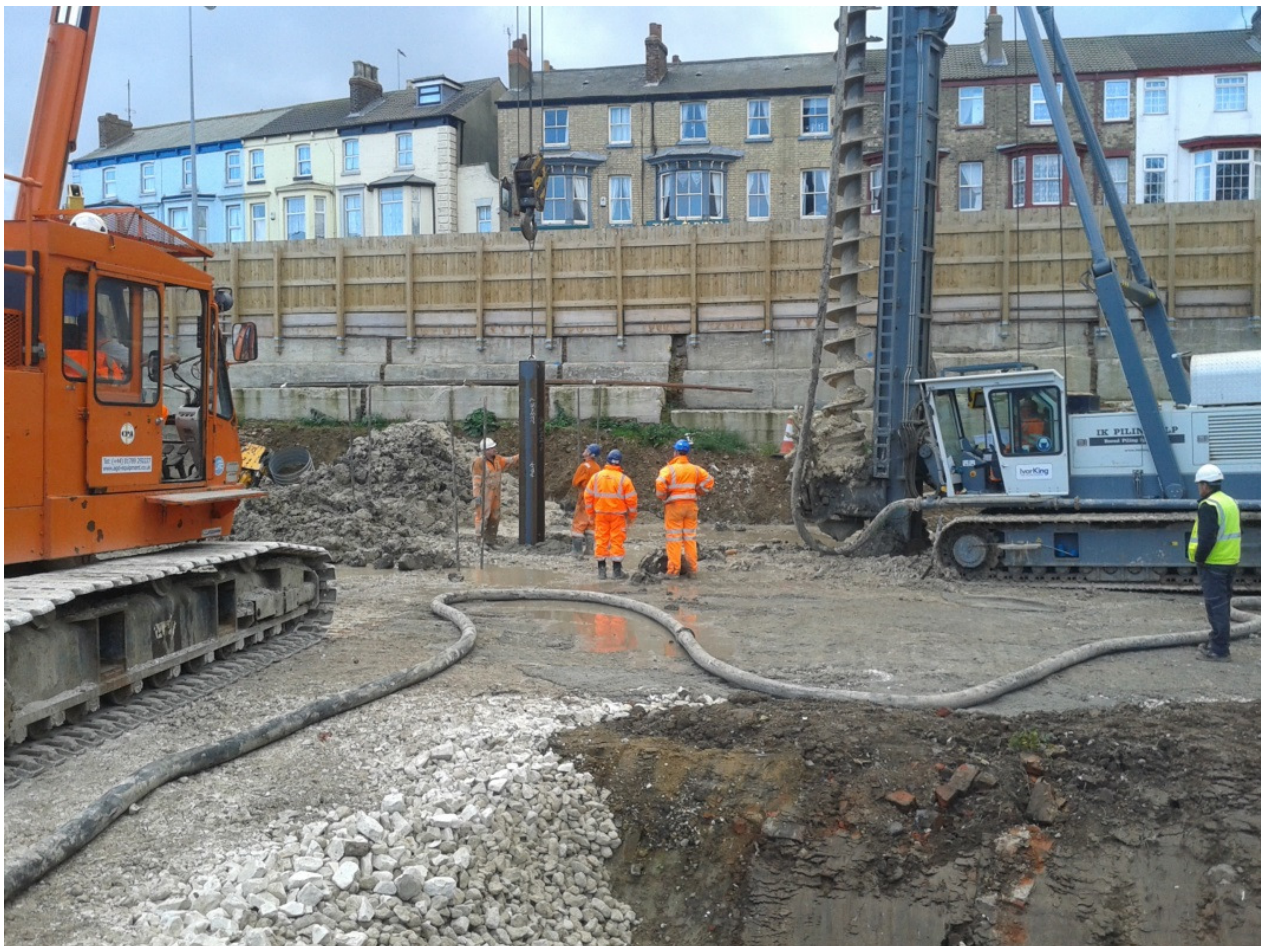
Beck Hill Piling Works
