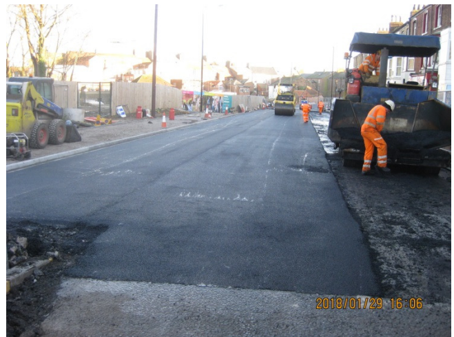
Laying the new road
